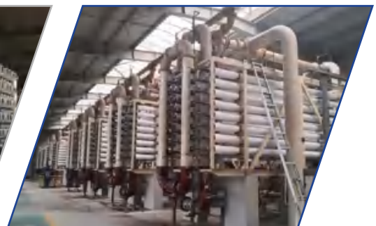
Dalian Hengli petrochemical water treatment project. Nov 2017
