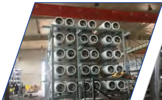
Daya Bay Cnooc's refinery project. July 2016
