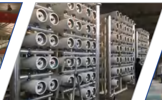
Qingdao wastewater reclamation project. Aug 2016
