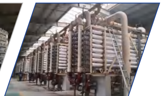
Dalian Hengli petrochemical water treatment project. Nov 2017
