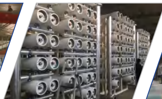
Qingdao wastewater reclamation project. Aug 2016
